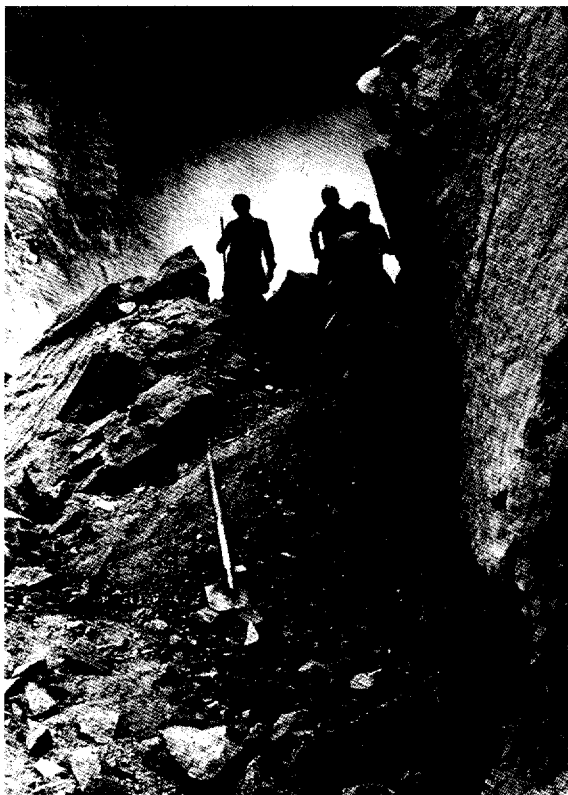
Fig. 43. The recent construction of the Aliabad irrigation channel which links the Hassanabad glacier with the fertile oasis of Central Hunza. The same rock-blowing and retaining wall construction techniques are used for building road tracks.
